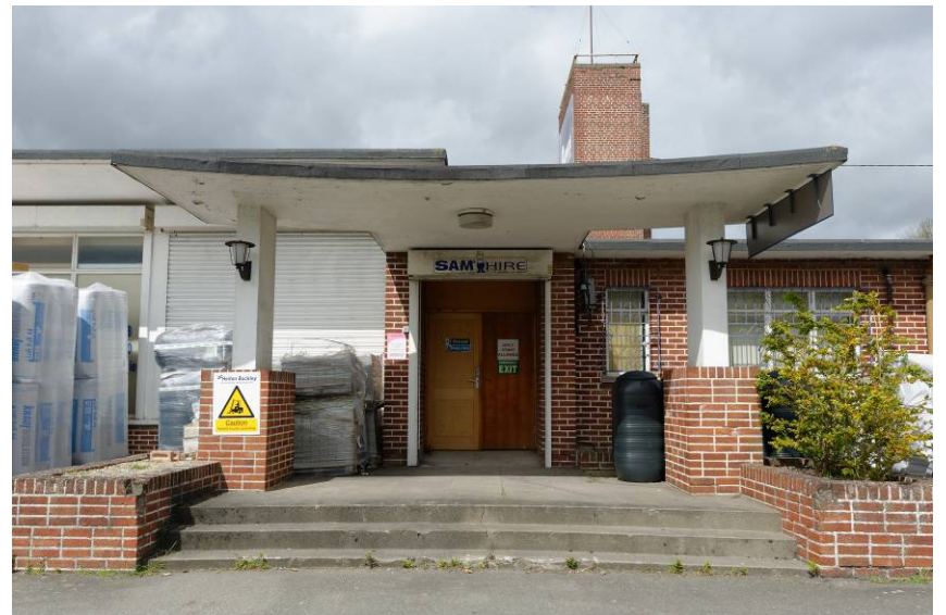
PIC 11; FREE-STANDING CANOPY OF (PRESUMABLY) IN-SITU CONCRETE.
